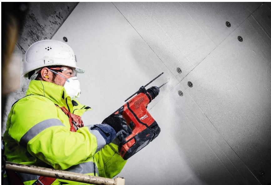
Fastening of pre-fabricated fire protection boards
